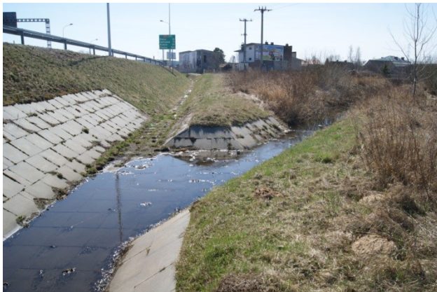
Phot. 4. Section IV – river bed of the Dulewie stream, near the S7 highway, functions as a collector of surface runoff waters
